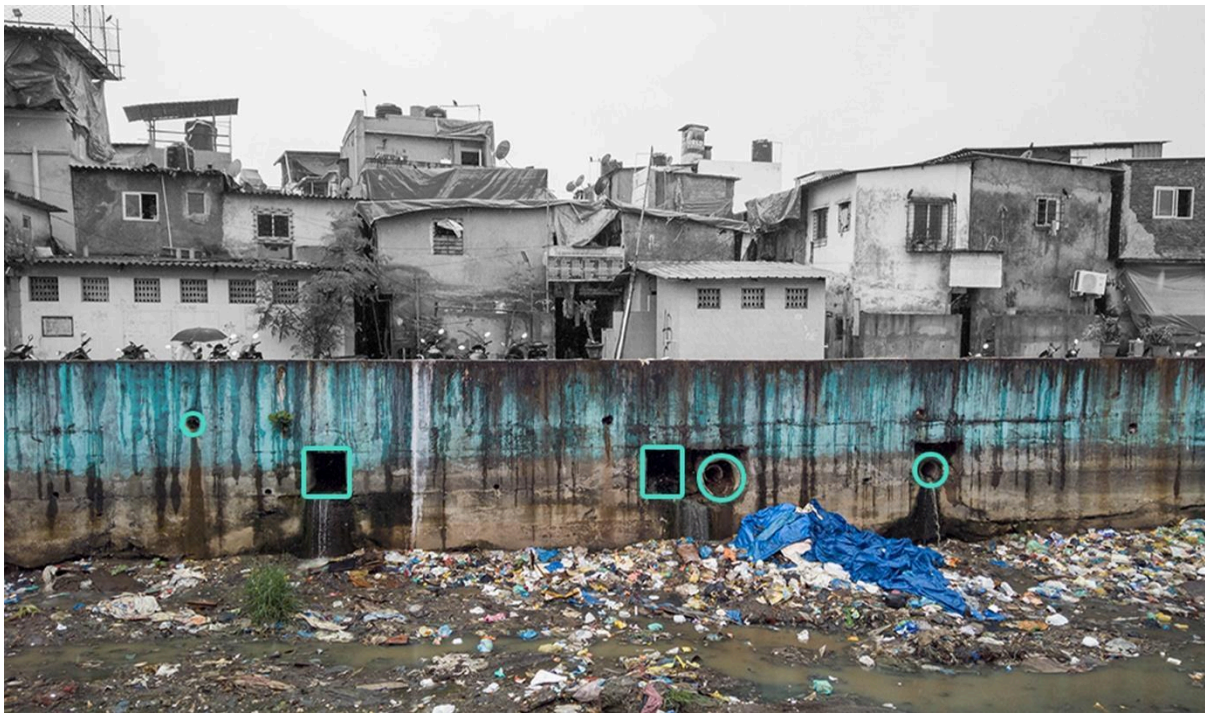
Fig. 3: Illegal Sewage lines connected to Nullahs (Source: Author)
